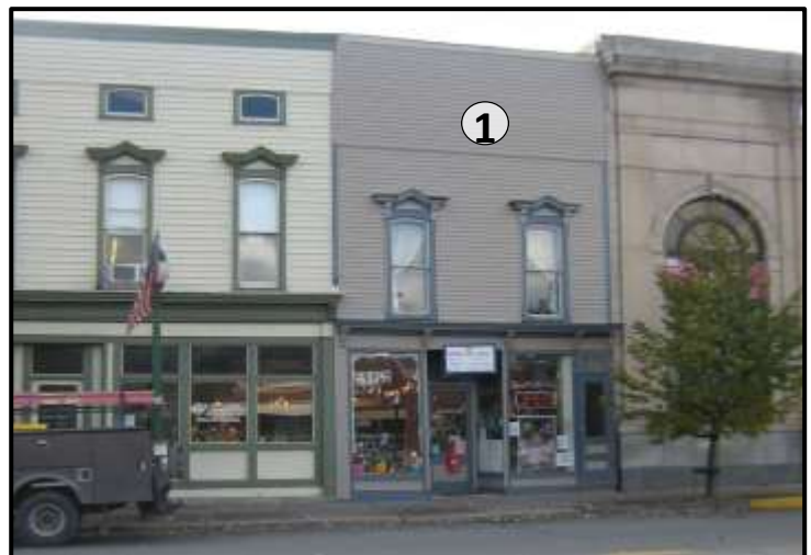
The image above demonstrates use of inappropriate materials and finishes (1). The materials used diminish the visual quality of the structure and adjacent buildings. In this example, although the structure has a high quality storefront, the use of a solid mass of vinyl siding with no vertical break over what was likely masonry construction reduces the overall appeal of the building.
