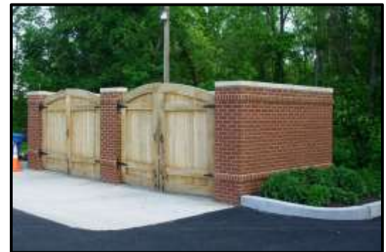
The above detached refuse enclosure is placed at the rear of the building and is composed of like materials as found in the principal structure.
