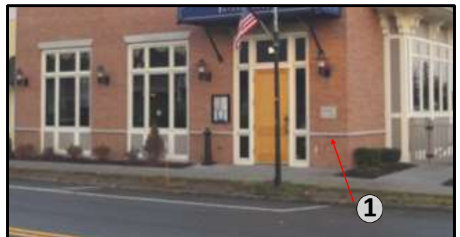
Although subtle (1), the highlighting of the building base anchors the structure to the site, and provides visual distinction between the ground plane and the structure. Material selection shall complement the architectural style of the building and those materials commonly found within the area.
