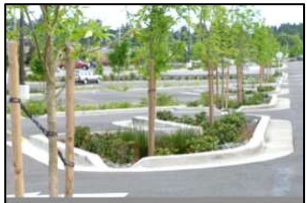
Where appropriate, bioretention areas and bioswales similar to the above may be used to promote the infiltration of storm water. These installations would be appropriate in parking lot medians or in linear strips along drive aisles or behind parking lots in lieu of large retention facilities.
