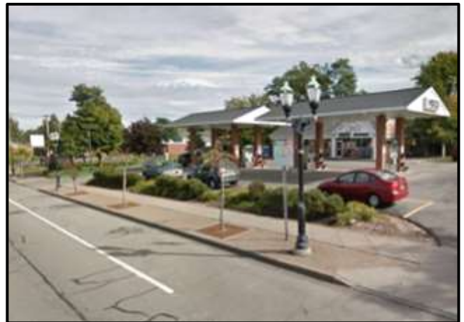
The image above features two separate fueling canopies, held by brick pillars. Vegetation is used to buffer the fueling station from sight for pedestrians and vehicles.
