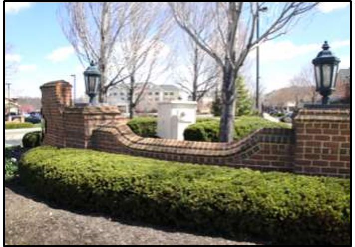
When required to be placed within view of the public, ground-mounted utility boxes should be screened or designed as an integral element within the site.
