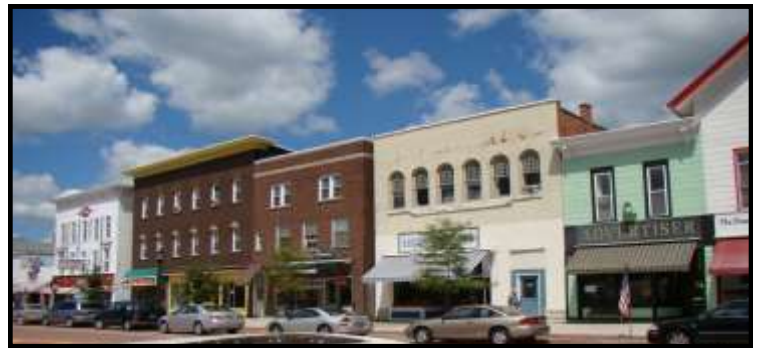
Enhanced transparency on store frontages, and the repetitive rhythm of the entryways creates a vibrant and active streetscape.
