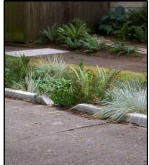
Efforts should be made to integrate storm water management into the numerous small greenspaces within the urban environment adjacent to driveways and parking lots, consistent with the most current New York State Stormwater Management Design Manual.
