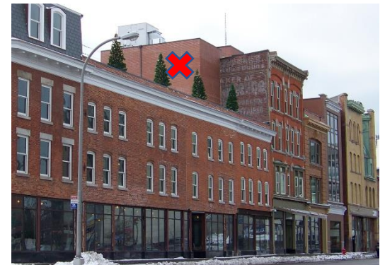
This elevator shaft addition extends two stories past the roofline, negatively impacting the historic character of the building.
