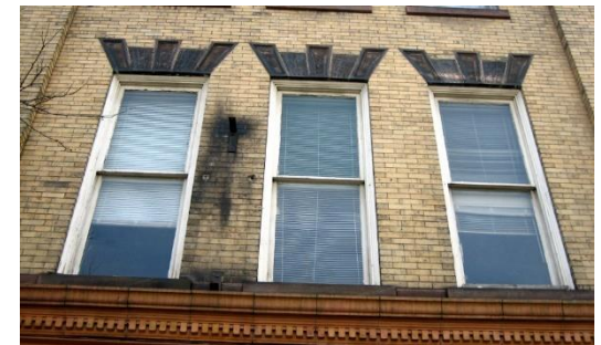
Before - Wood windows deteriorated beyond use.
