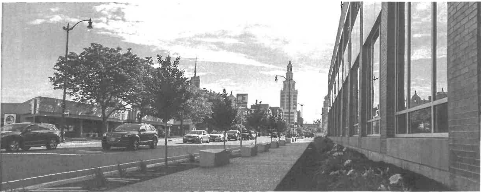
/ Green infrastructure planters and street trees installed along Genesee Street
